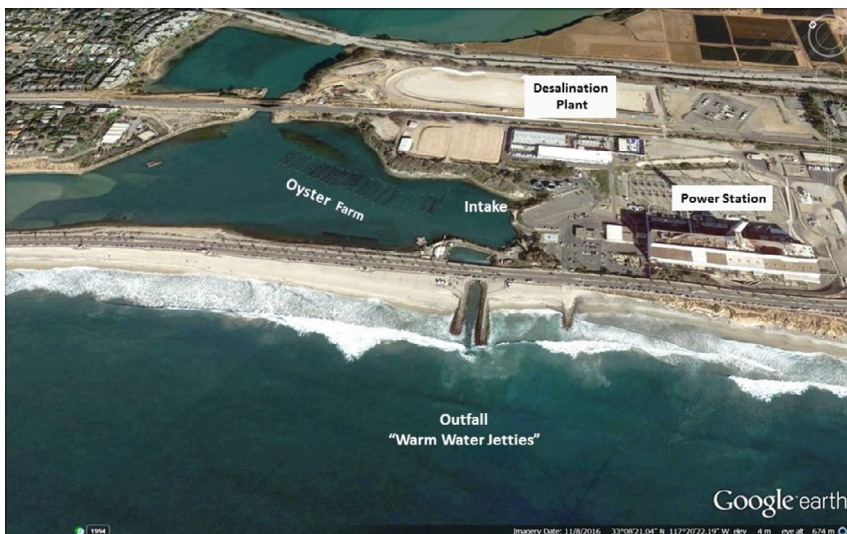
Fig. 14.1 Carlsbad, California desalination facility, operated by Poseidon Resources, Inc. Colocated with and using inflow/outflow infrastructure of an existing power plant. Residential neighborhoods are located in upper left across the Agua Hedionda Lagoon. The public has access to the beach located across the coastal highway. Source: Google Earth, 33°08' 21.04" N and 117°20' 22.19 W (11/8/16).
